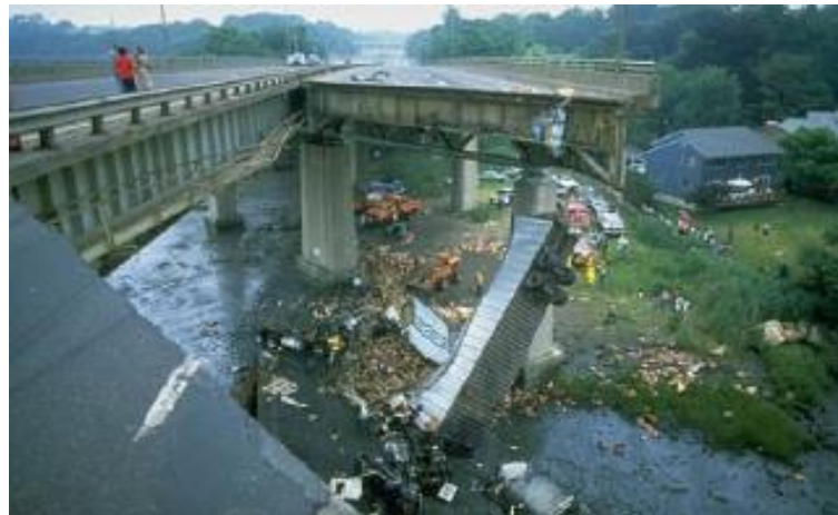
Collapse of the Mianus River Bridge
