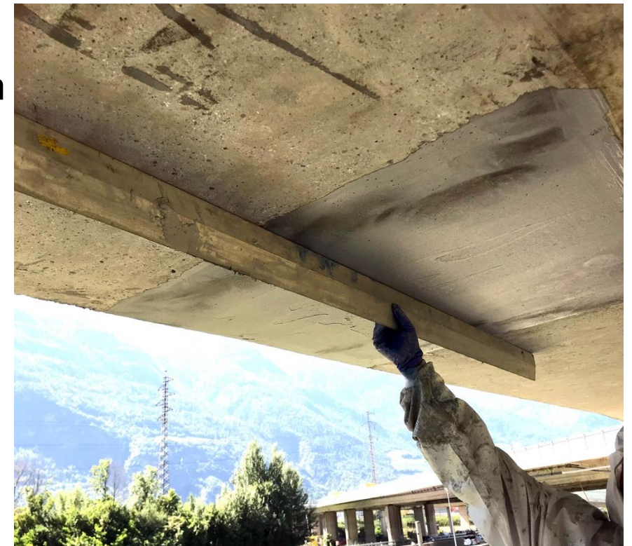
S&P reinf., bridge Riddes, 2021
